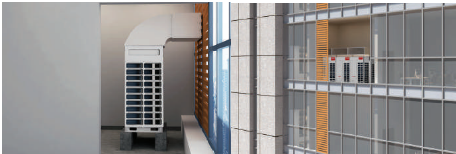
Installation of duct
